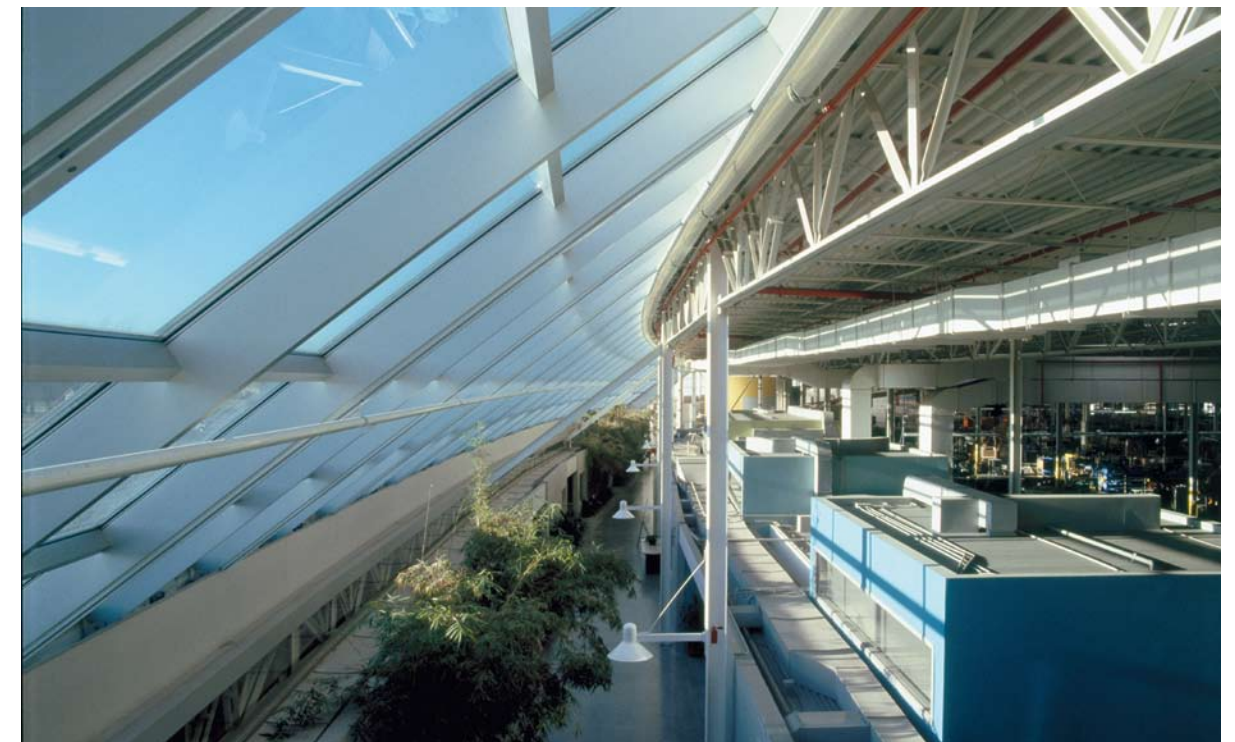
THE HERMAN MILLER GREENHOUSE MANUFACTURING AND OFFICE BUILDING IN HOLLAND, MICHIGAN, WAS A PILOT FOR THE DEVELOPMENT OF LEED CERTIFICATION GUIDELINES, AND EARNED "PIONEER" STATUS FROM THE U.S. GREEN BUILDING COUNCIL.
