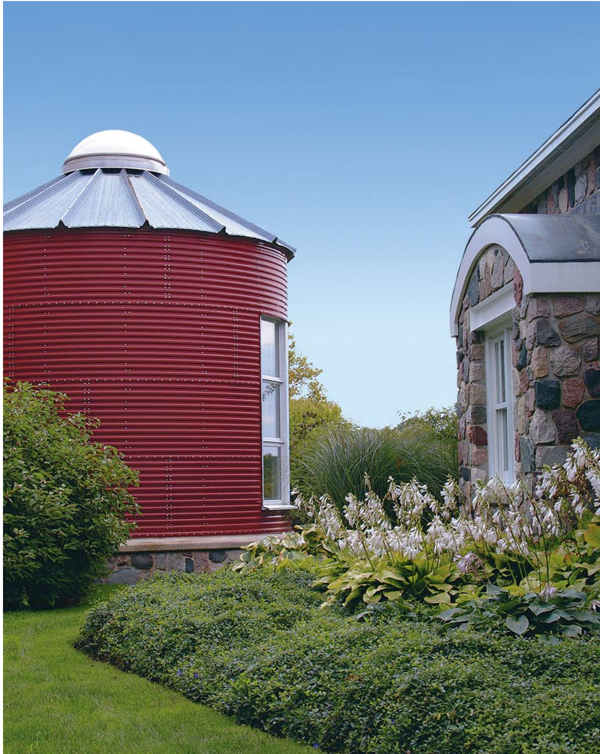
HERMAN MILLER'S DESIGN YARD FRONT DOOR IN HOLLAND, MICHIGAN, IS LEED GOLD CERTIFIED FOR COMMERCIAL INTERIORS.
